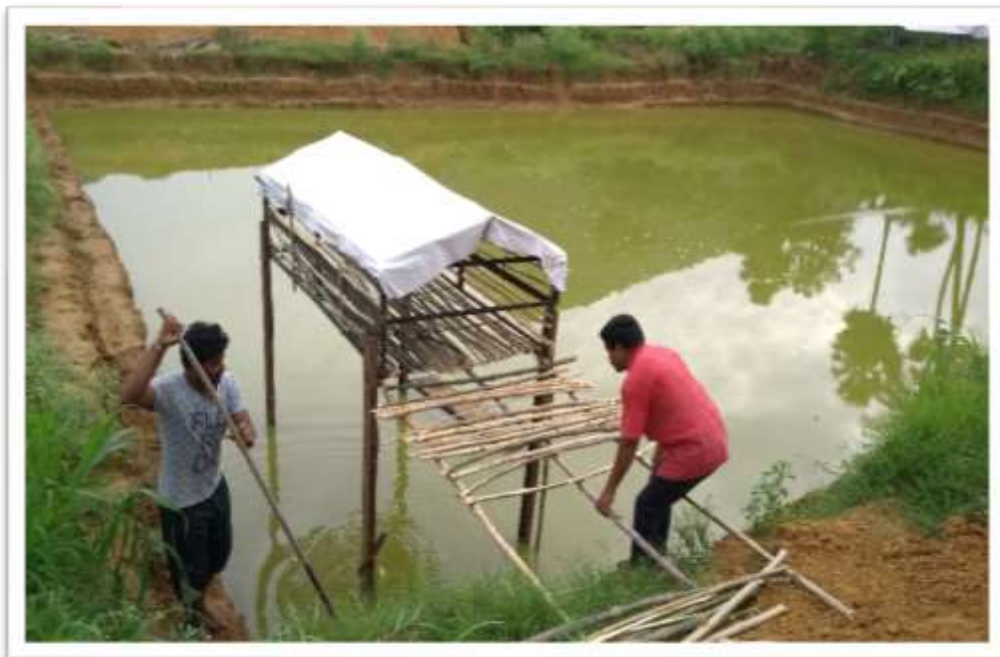
Poultry Shed Construction
